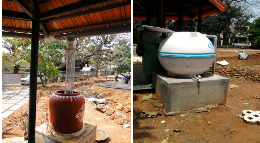
Plate 1: Rooftop RWH, Theme Park, Photo: Manasi. S
